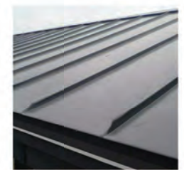
Aluminium Standing Seam Roof
